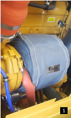
PHOTOS 1-4 PHOTOS 5-7 Cat 24 manifold, turbo, e/pipe, muffler, t/pipe blankets
